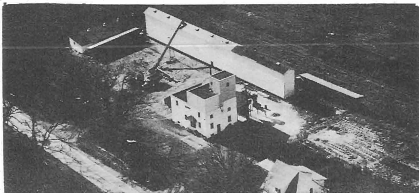
MANLEY ELEVATOR NO. 3—MIDDLEBURY, INDIANA
